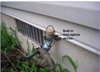
The interior cutoff for the hose bibbs were located. These should be turned off in winter and drained to prevent freezing.
